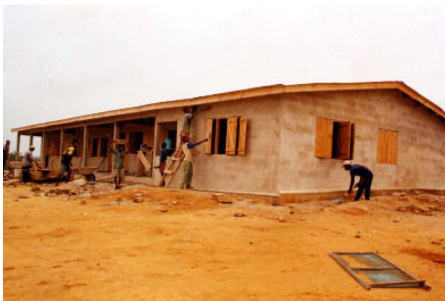
The secondary school in Shama-Kedzi in its advanced state of construction.
