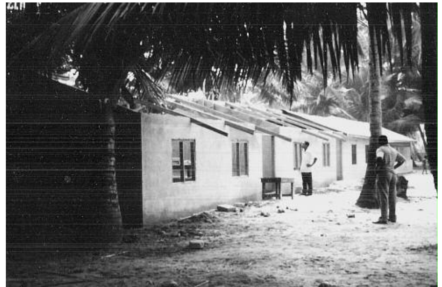
Construction of Abakam school in good progress
